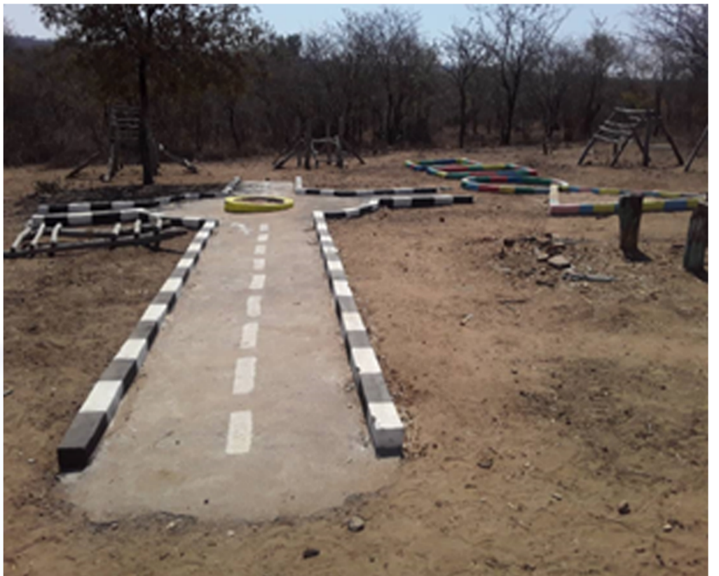
Completed outdoor play area
